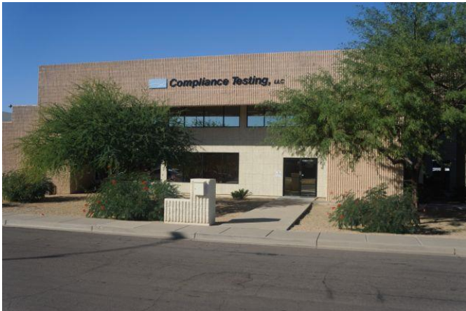
Meeting Site - Compliance Testing, LLC in Mesa, AZ.
